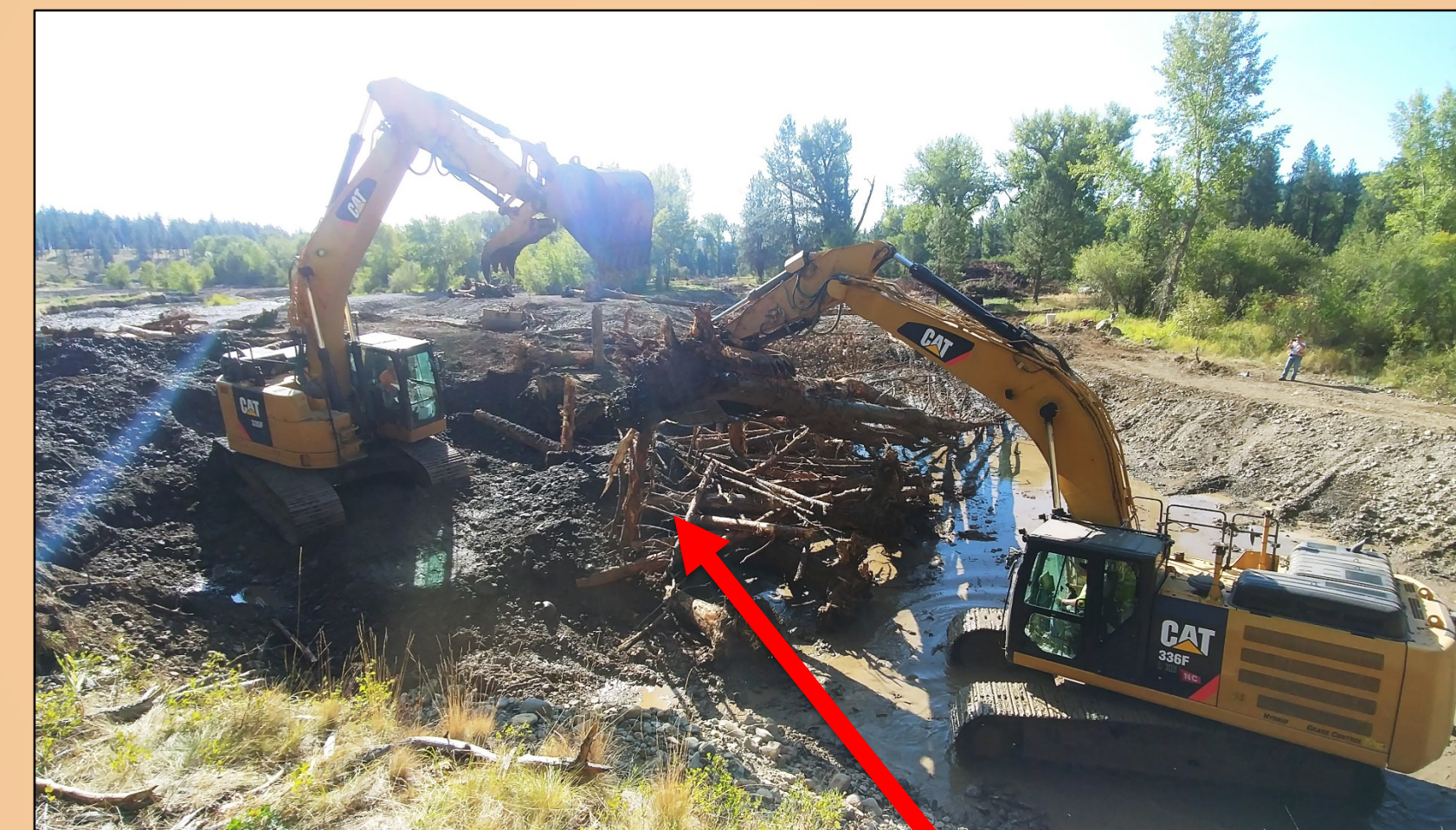
Large wood structure construction at station 42+00, August 23, 2019 (looking downstream).
