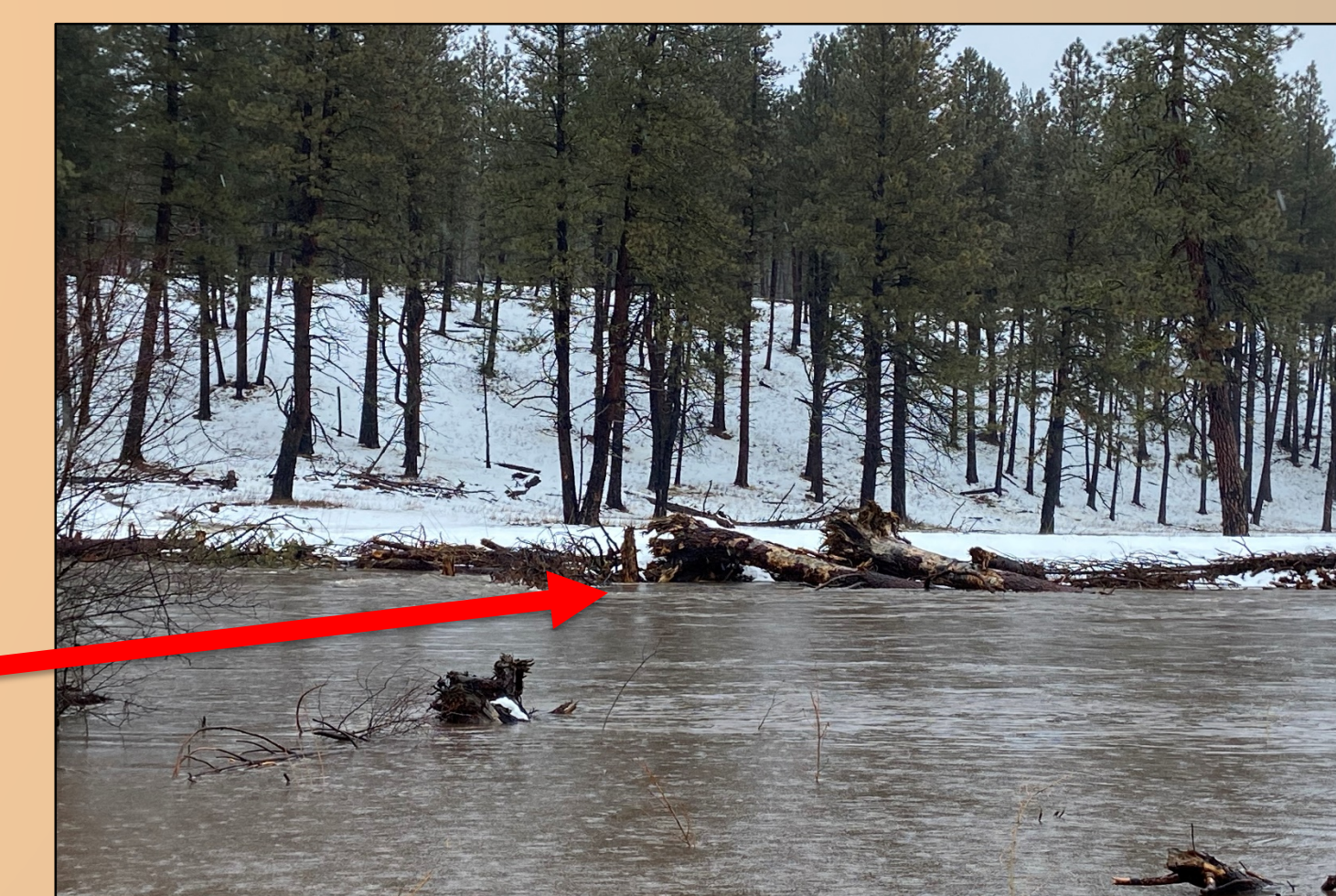
Large wood structures at station 42+00
