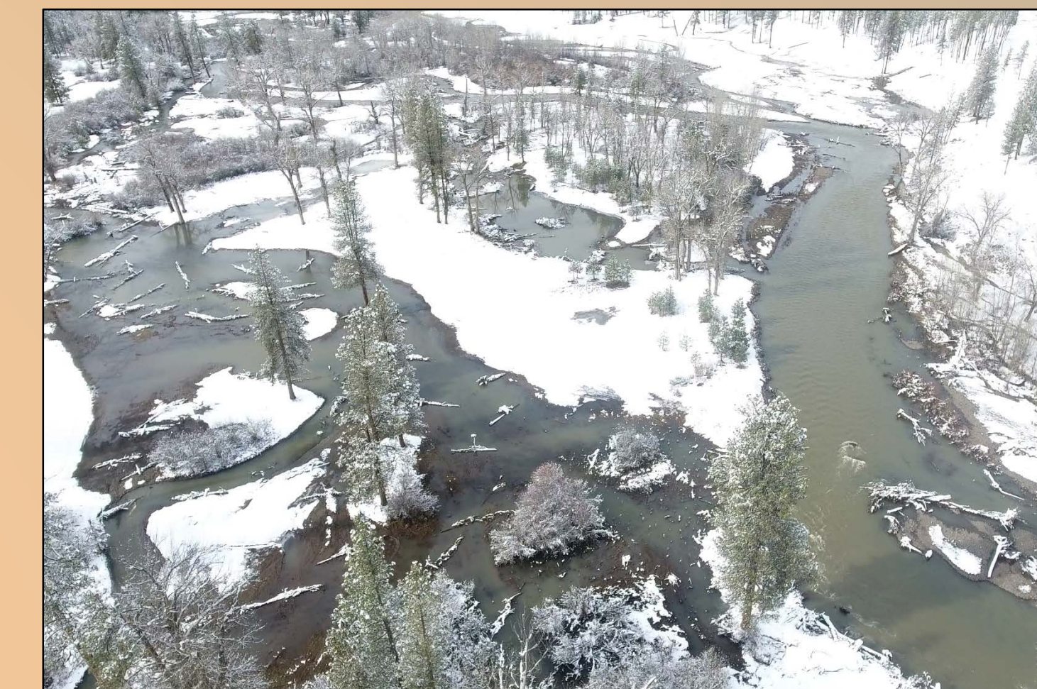
Floodplain activation at station ~80+00
