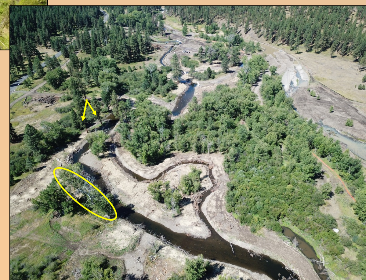
Main channel and side channel 5 post-project, looking upstream
